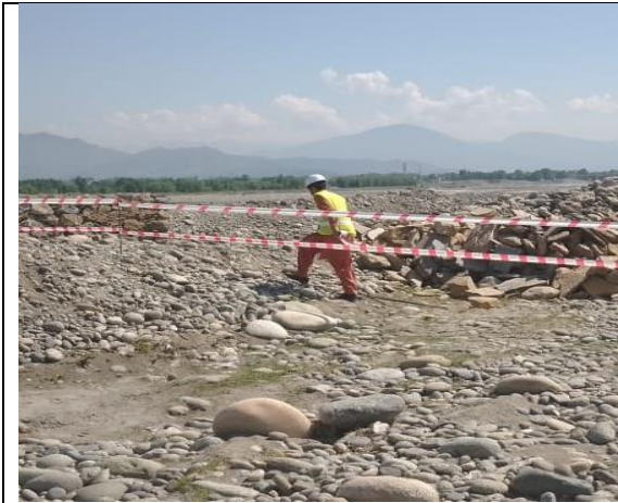
Workers wearing PPEs at Jalwanan Site
