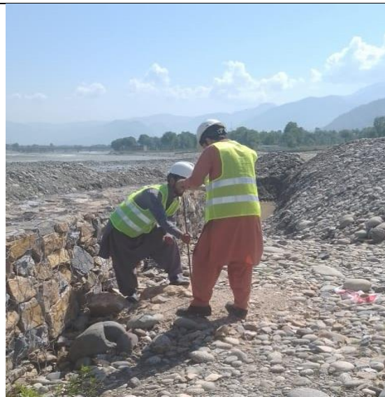
Workers at Asala Site (Package 13 Scheme 2)
