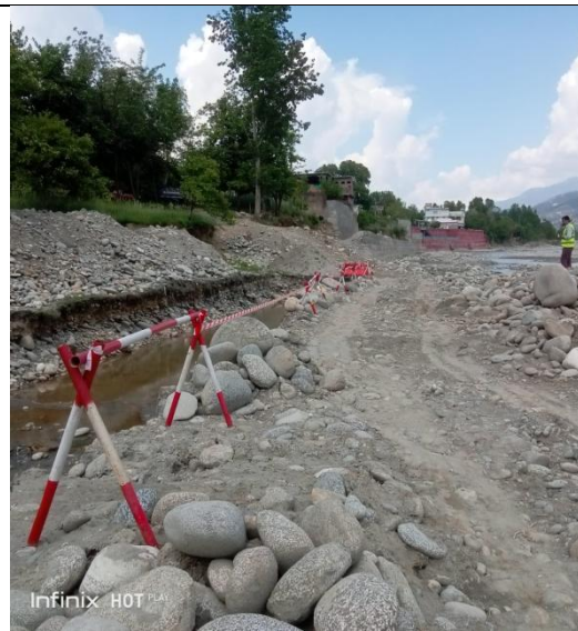
Barrage at Dakorak (Package 13 Scheme 1)
