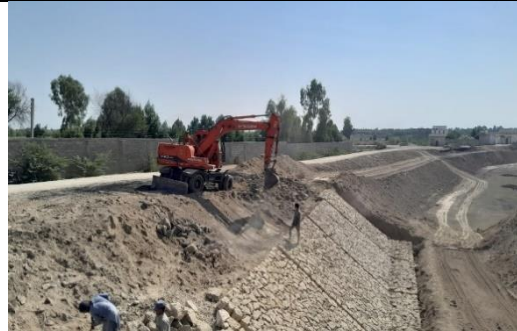
Ongoing Construction Activity at FCC 03, Package 5
