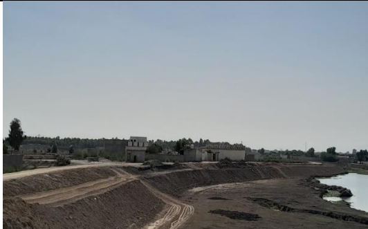
Ongoing Activity at CRBC, Package 3
